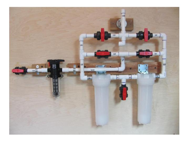
Wet 0-rings on top of the 25mm or 10 inch filters and insert up into Filter Mount Assembly.
