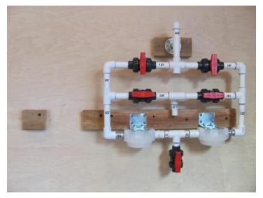
Bolt wooden supports to the wall spacer removed.
